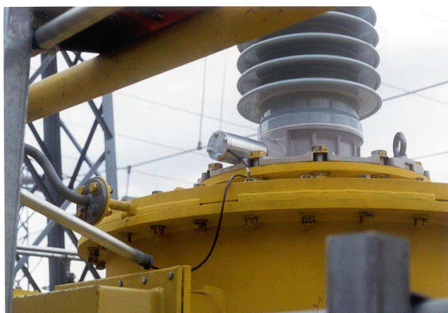
Fig. 7 PD sensor at bushing capacitance tap
